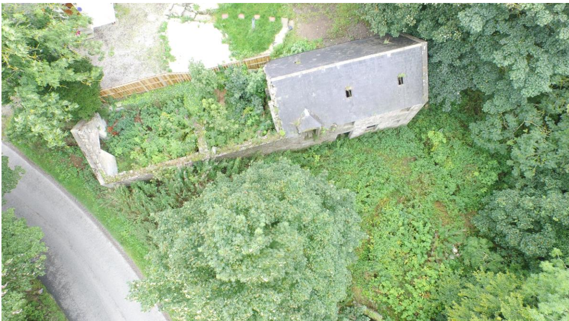
Aerial view of the existing building and woodland
